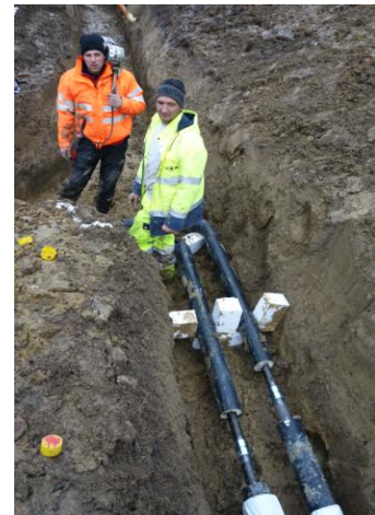
Pressfitting installed
