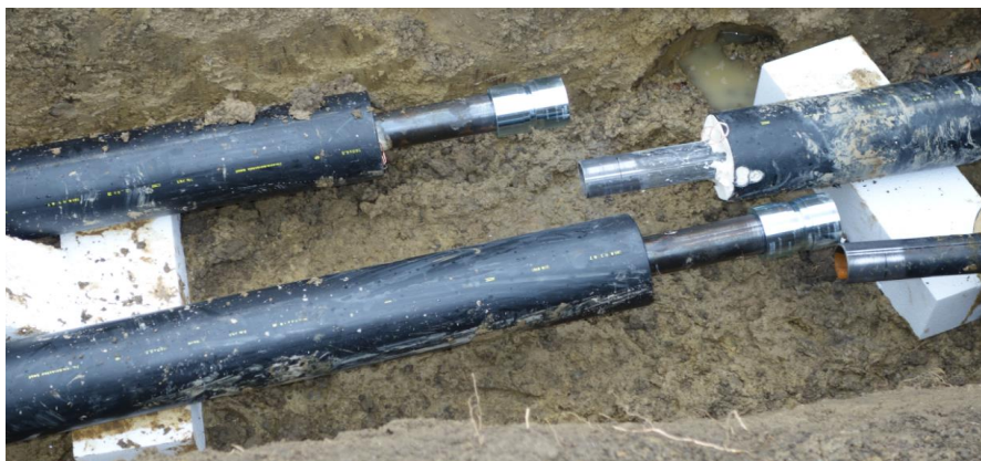
One side of the fitting is pressed. Then the other side of the tube is inserted.
