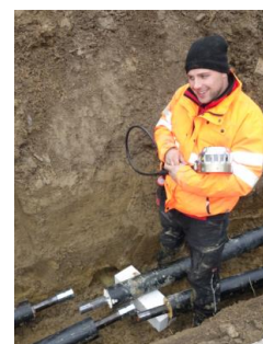
Construction worker holding press tool
