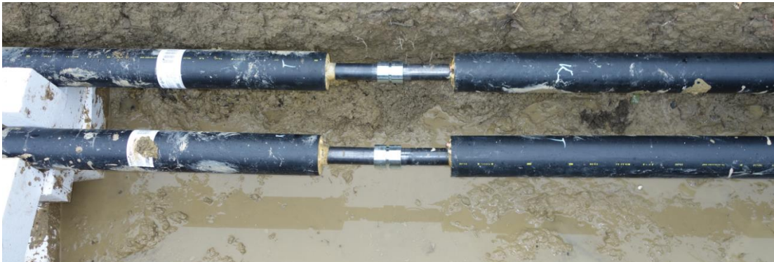
Pressed fittings flow- and return line during pressure test
